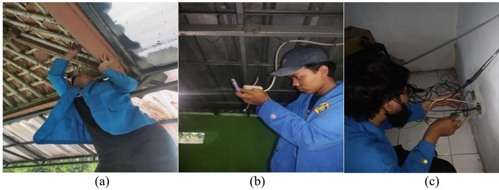
**Gambar 4.**(a) pergantian kabel (b) pergantian fitting lampu (c) pergantian stop kontak
